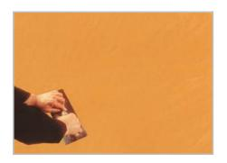
Step 5 - When the product begins to dry, proceed with compacting and polishing the wall.
